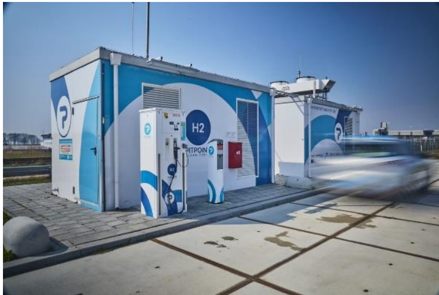
Figure 21. Groningen's Hydrogen Refueling Station (HRS) with a car dispensing unit @700 bar [56]
